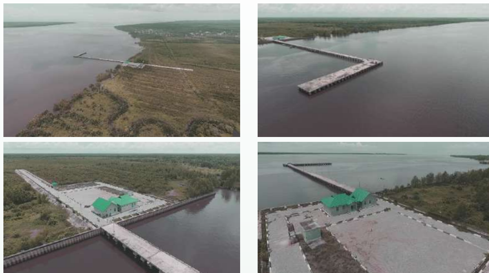
Gambar 4.3 Kondisi Pelabuhan Batanjung Figure 4.3 Batanjung Harbor Condition
