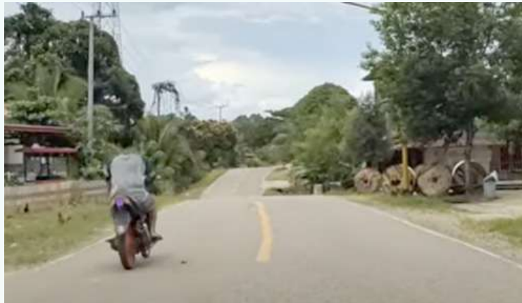
Gambar 4.12 Kondisi Jalan Trans Kalimantan di Teweh Baru Figure 4.12 Trans Kalimantan Road Condition in Teweh Baru
