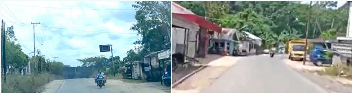
Gambar 4.20 Kondisi jalan di Teweh Baru | Figure 4.20 Road conditions in Teweh Baru
