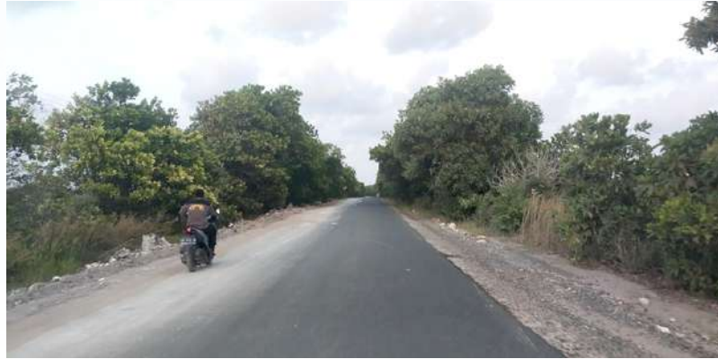
Gambar 4.22 Jalan poros Sukamara - Pantai Lunci - Jelai | Figure 4.22 Sukamara - Pantai Lunci - Jelai axis road
